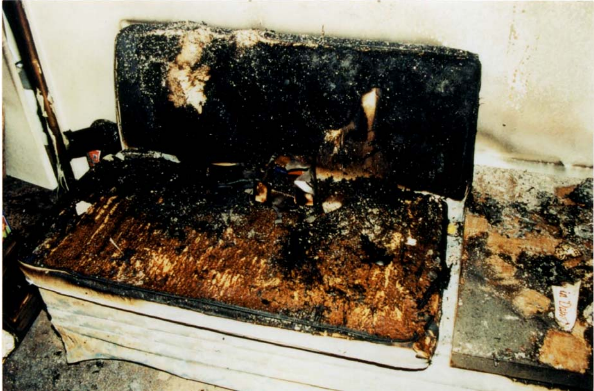
Figure 73: Unlike the Back of the Couch, the Front Shows Clear Evidence of Burning
