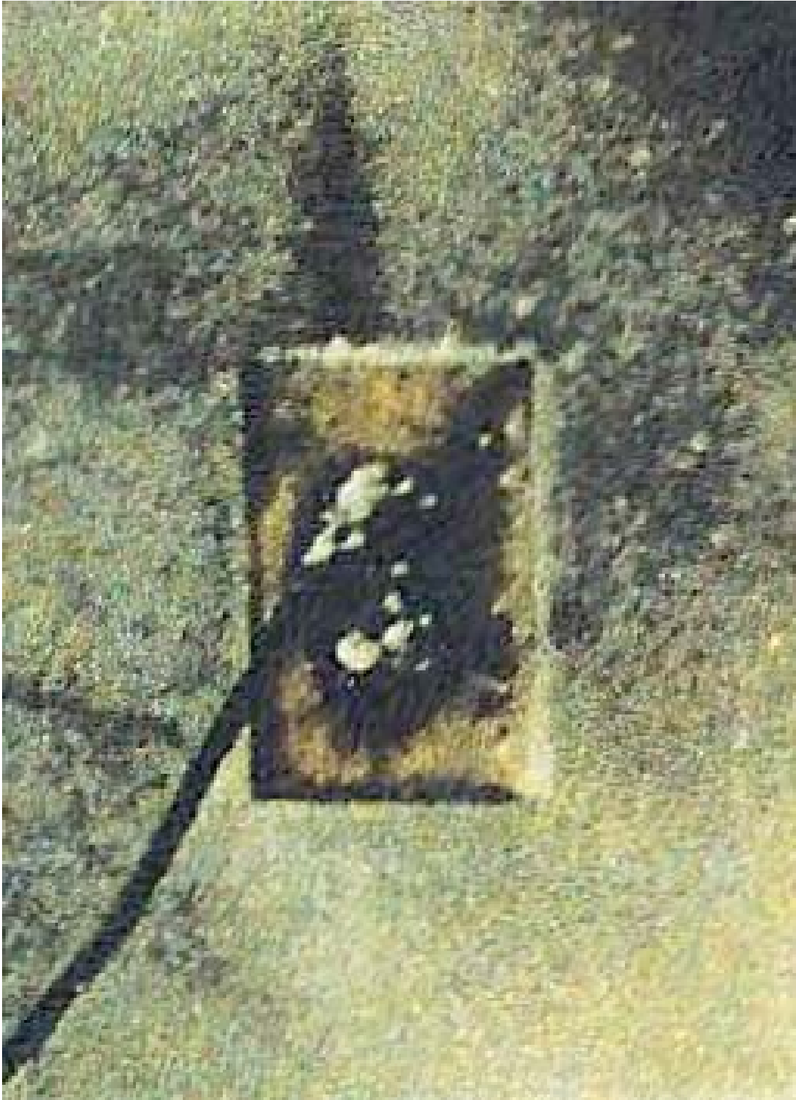
Figure 1: Smoke Streaks Reveal Fire Within Electrical Outlet
