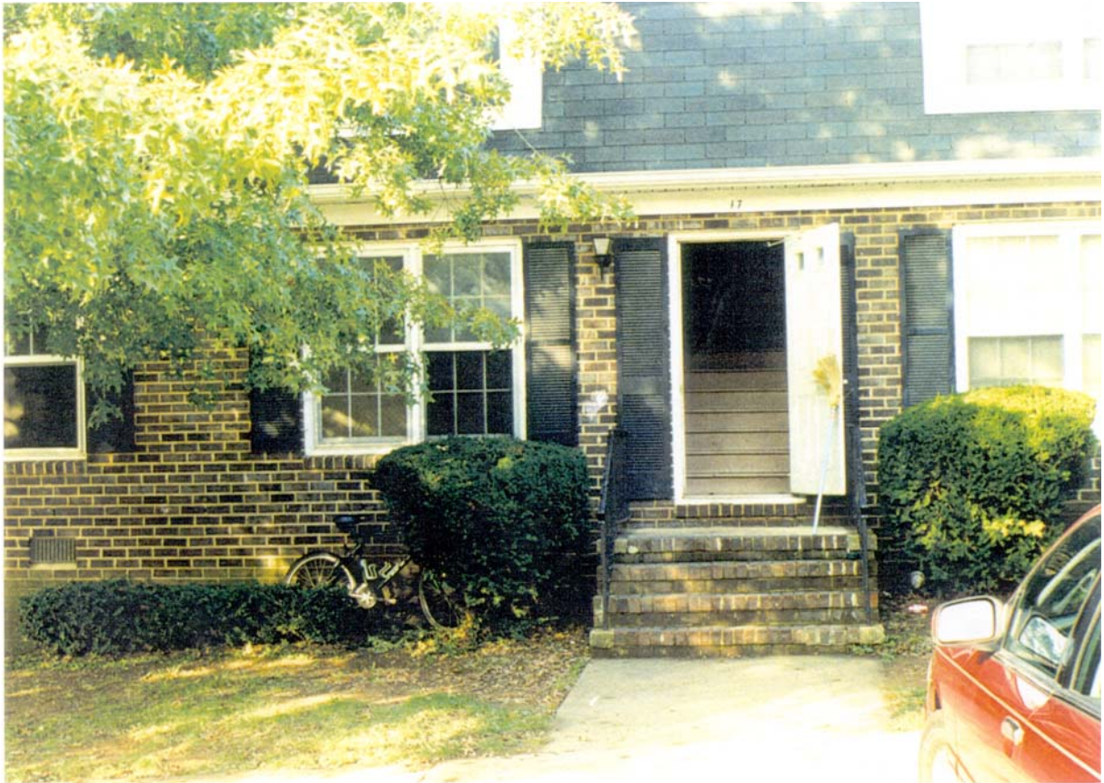
Figure 7: Entry of Building 17 -- Ledford Apartment on Left
