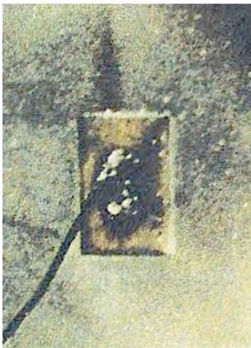
Figure 74: Faceplate and Front Door Chime Each Reveal Fire from Behind
