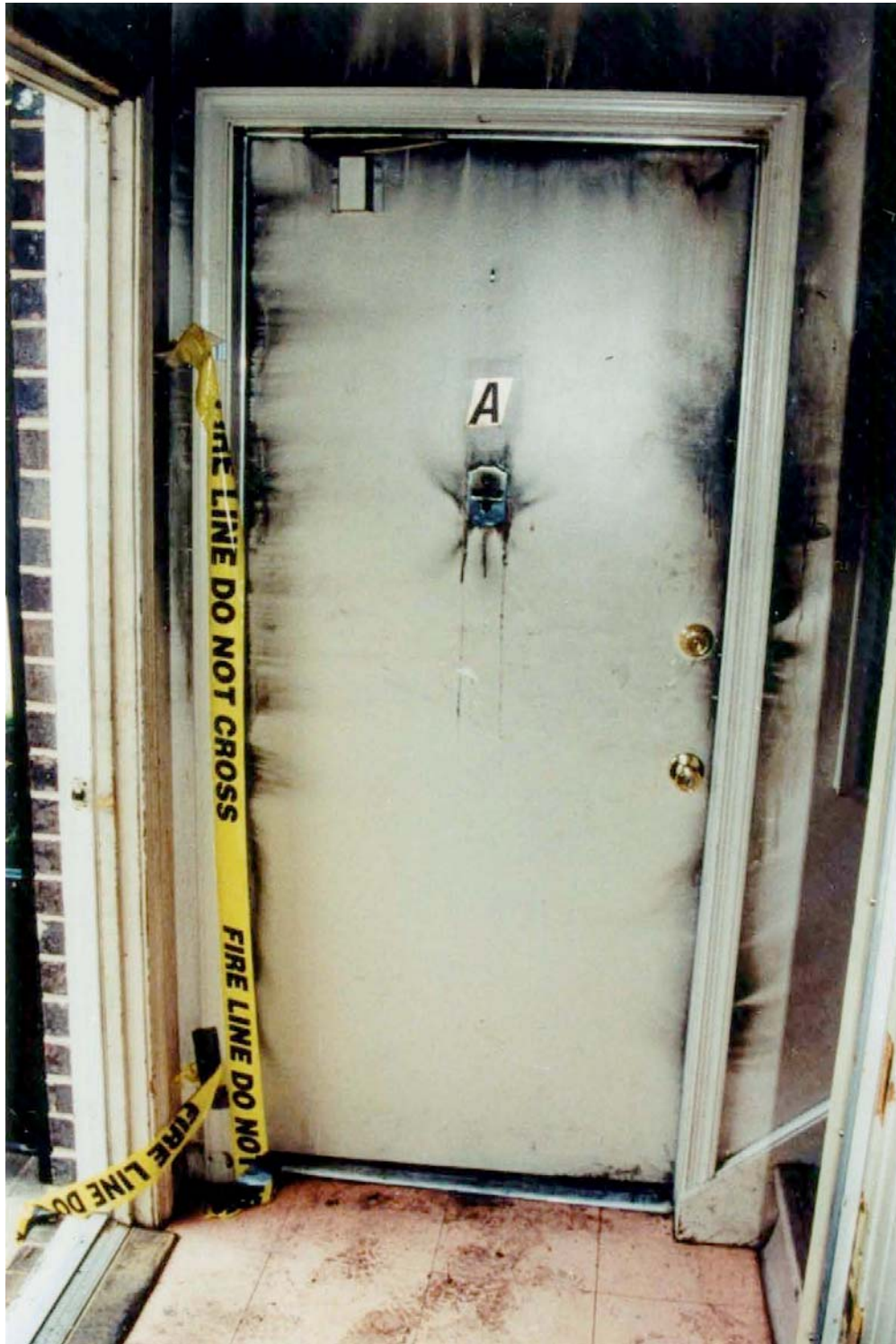
Figure 8: Smoke Streaks Reveal Fire Within Apartment
