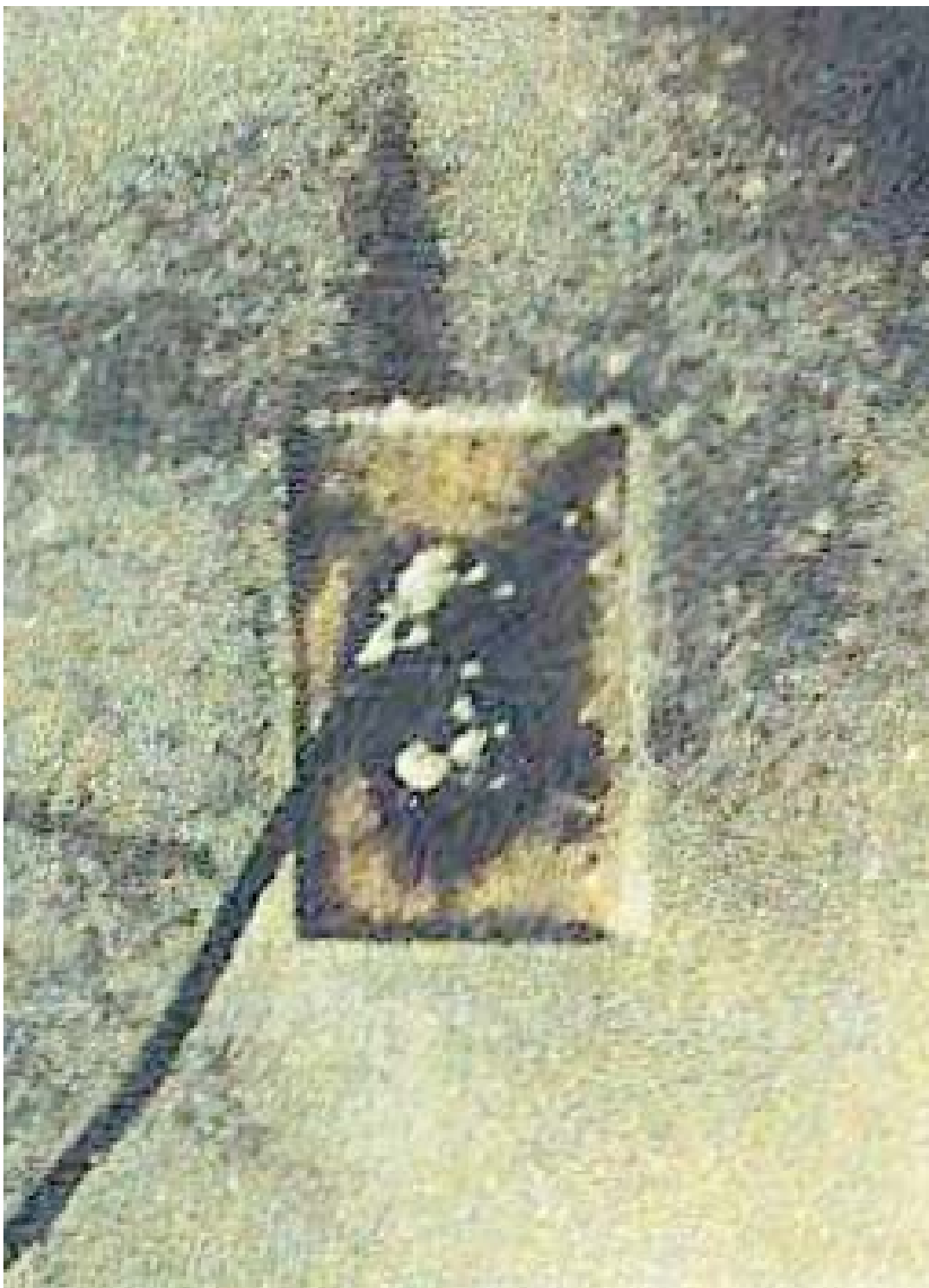
Figure 9: Smoke Streaks Reveal Fire Without Electrical Outlet
